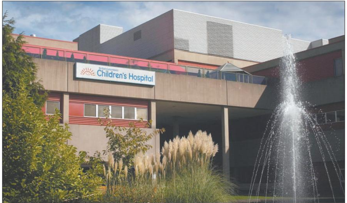
Work on B.C. Children's Hospital in Vancouver is to be completed by 2014. JON MURRAY FILE PHOTO — THE PROVINCE
